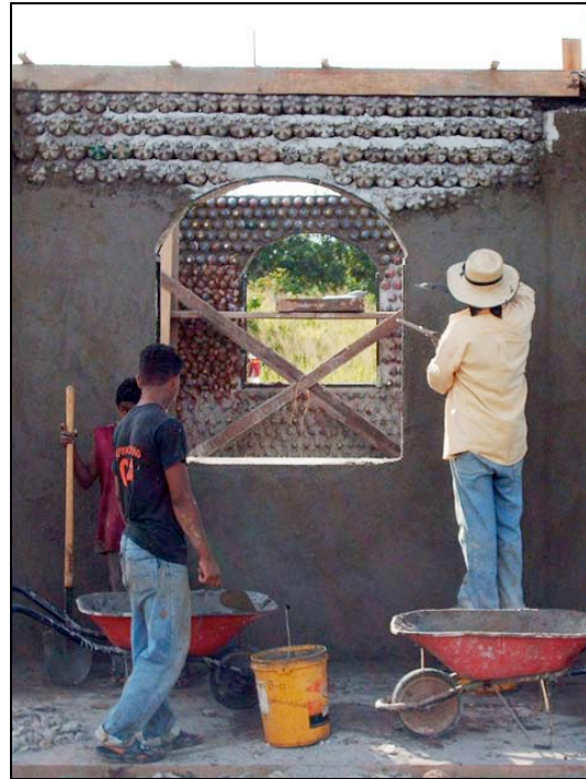
and plaster the walls.
